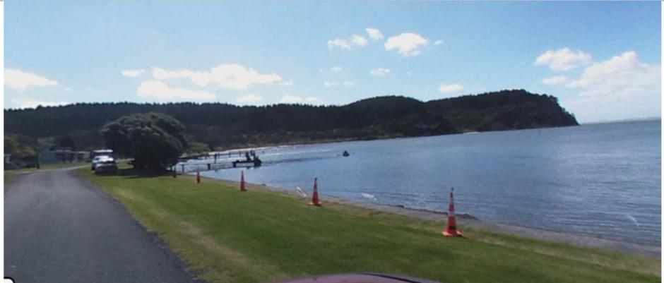
View south east on boat ramp - note insitu mass concrete pours for bank erosion protection either side of ramp
